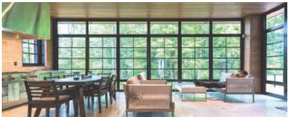
WeatherMaster® V4T Windows Installed in Existing Structure
